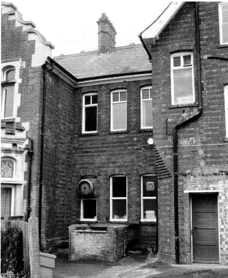
Fig. 8 (left) Typical Seckham brickwork and windows surviving on the north elevation of the Mansion, with Leon's Dining Room addition of c.1906 on the far left © English Heritage. NMR, DP003682.jpeg
